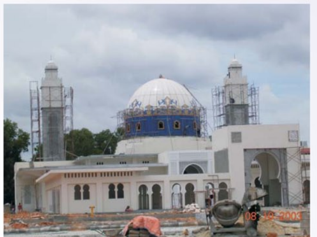
◆ INSTALLATION OF COMPOSITE PANEL AND TOUCH - UP PANEL JOINT
