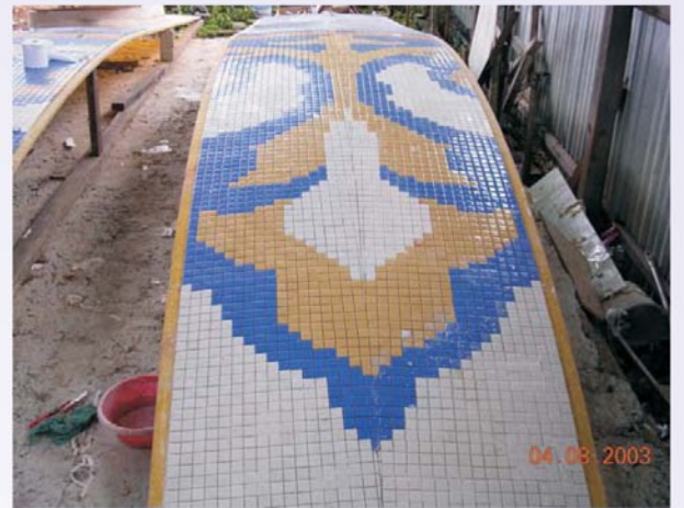
◆ COMPLETE LAYING OF MOSAIC FOR ONE SEGMENT
