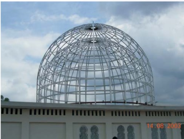
◆ ERECTION OF ALUMINIUM STRUCTURE
