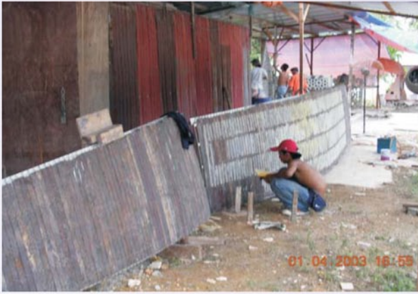
◆ PREPARATION OF ALUMINIUM MOULD
