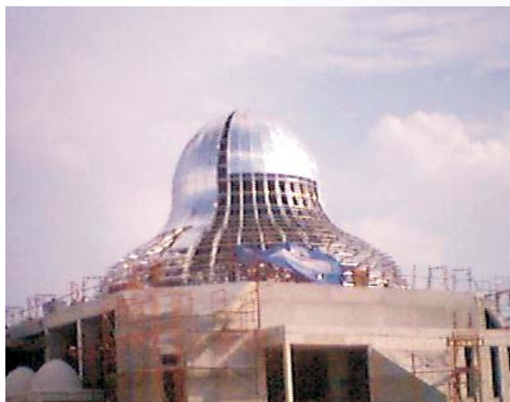
◆ INSTALLATION OF ALUMINIUM WATER PROOFING LAYER
