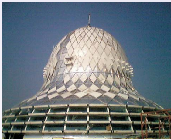
◆ INSTALLATION OF EXTERNAL ALUMINIUM SOLID PANEL
