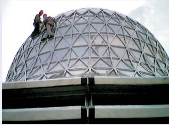
◆ INSTALLATION OF EXTERNAL ALUMINIUM SOLID PANEL
