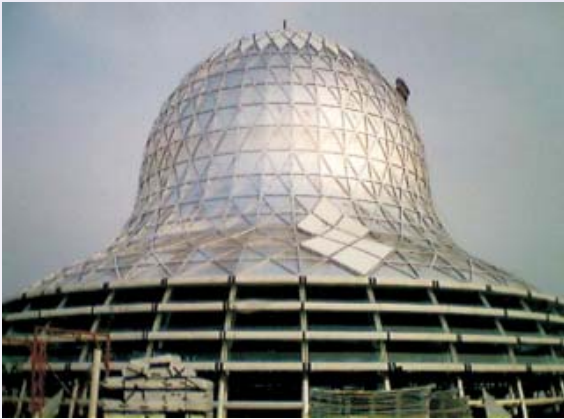
◆ INSTALLATION OF EXTERNAL ALUMINIUM SOLID PANEL
