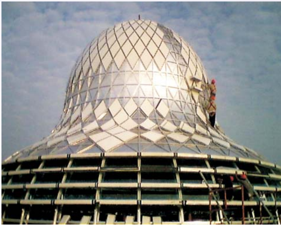
◆ INSTALLATION OF EXTERNAL ALUMINIUM SOLID PANEL
