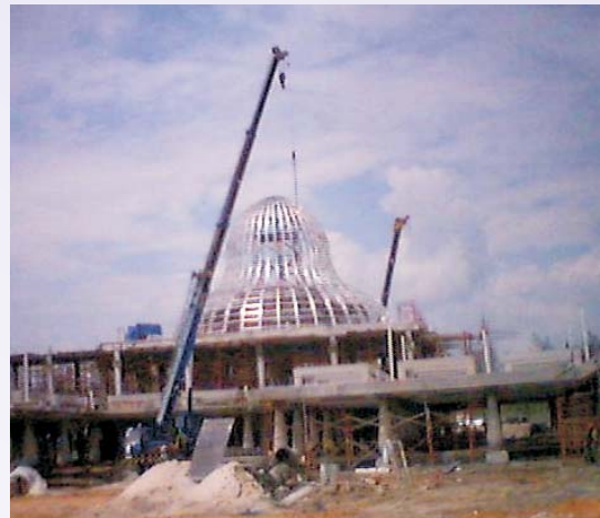
◆ ERECTION OF ALUMINIUM STRUCTURE
