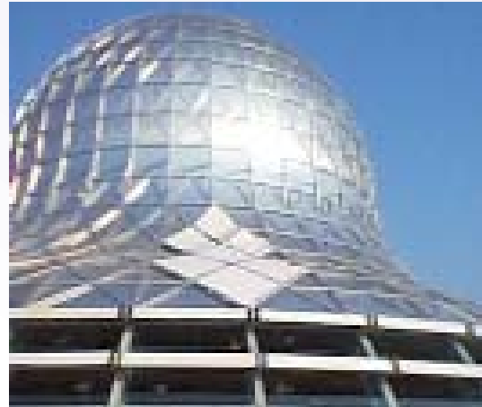
◆ INSTALLATION OF ALUMINIUM SUB-FRAME
