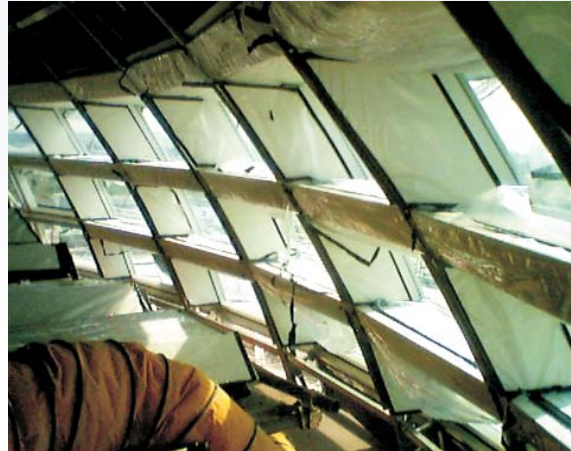
◆ INSTALLATION OF GLASS PANEL
