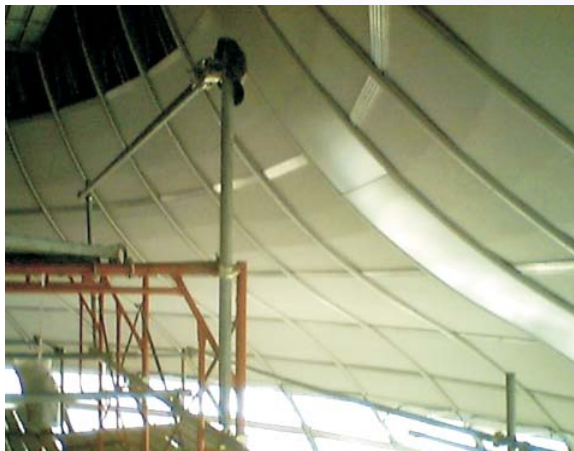
◆ INSTALLATION OF ACOUSTIC PANEL INNER DOME CEILING
