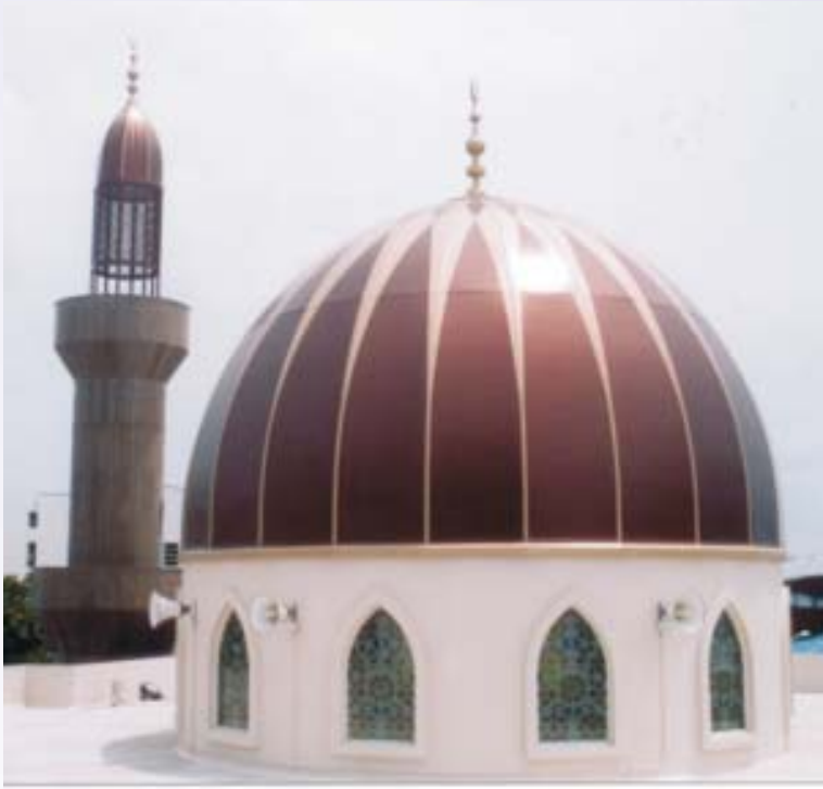
DESIGN, SUPPLY AND INSTALLATION OF ALUMINIUM DOME
