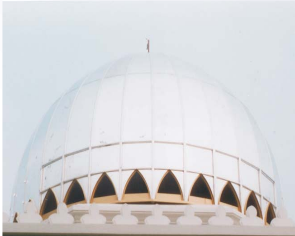
◆ INSTALLATION OF ALUMINIUM WATER PROOFING LAYER
