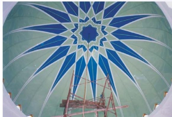
INNER ALUMINIUM DOME CEILING
